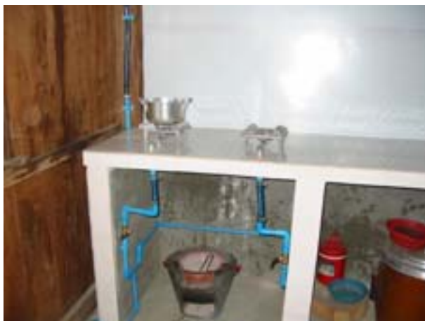
Fig 19: Installing gas burner
