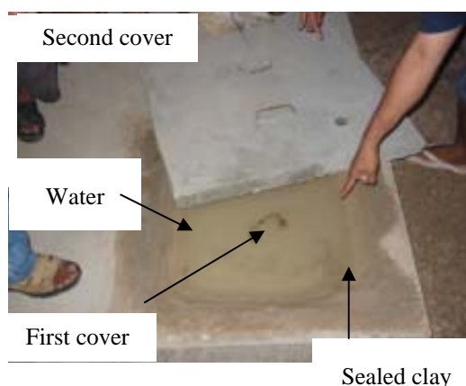
Fig 10: Technical hole and its two covers
