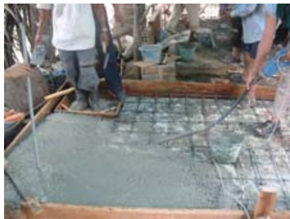
Fig 9: Vibrating concrete
