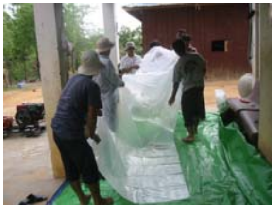
Fig 16: Assembling two plastic layers for gas reservoir
