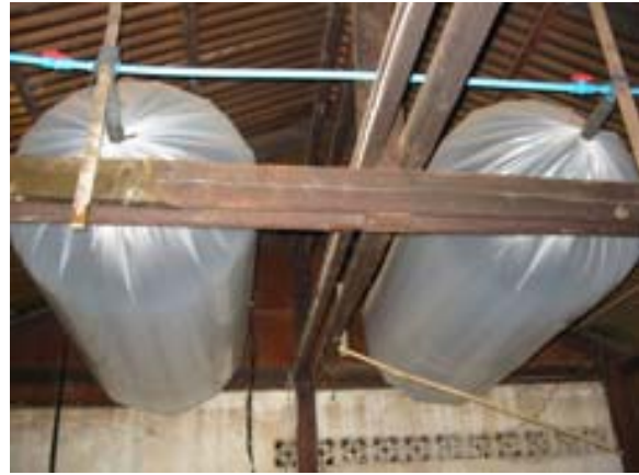
Fig 18: Double gas reservoir
