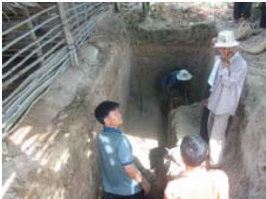
Fig 1: Digging digester hole and underground
