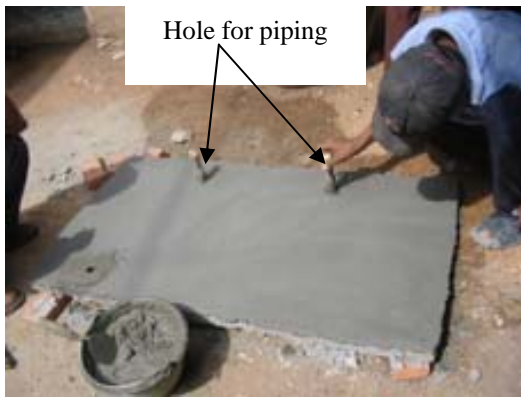
Fig 11: Plan and construction of worktop for cooking
