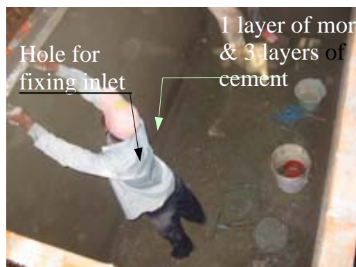
Fig 4: Plastering mortar inside the tank to protect leakage
