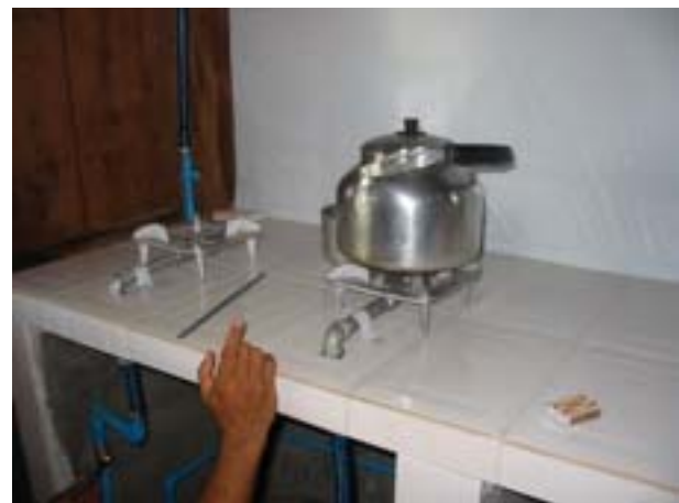
Fig 19: Installing gas burner
